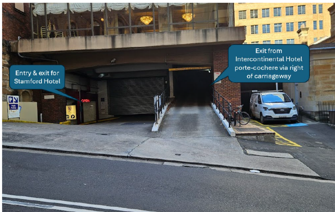
Figure 3 Existing vehicle egress from right of carriageway
