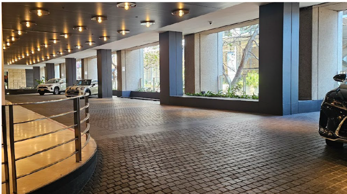
Figure 6 Existing porte-cochere servicing the Intercontinental Hotel
